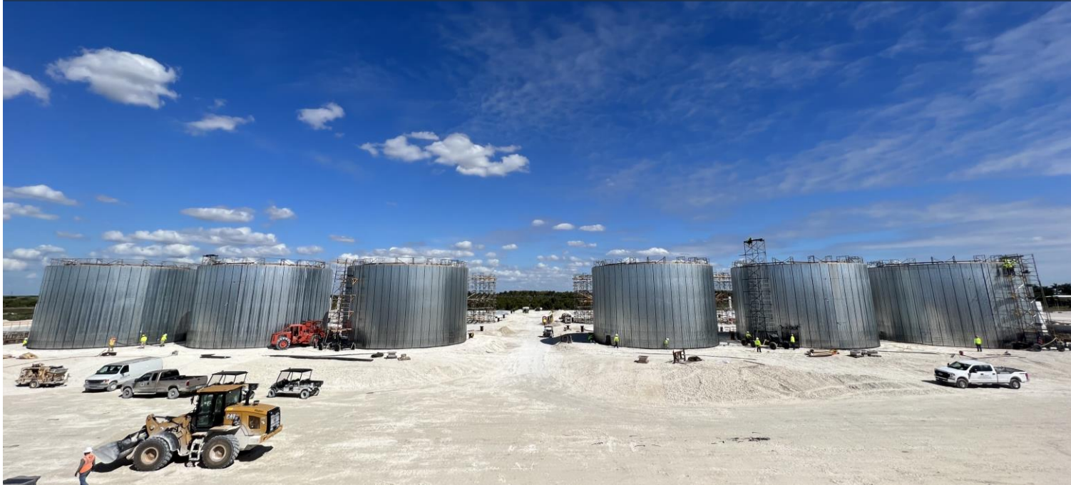
Phase 2 tanks (Mar '22)
