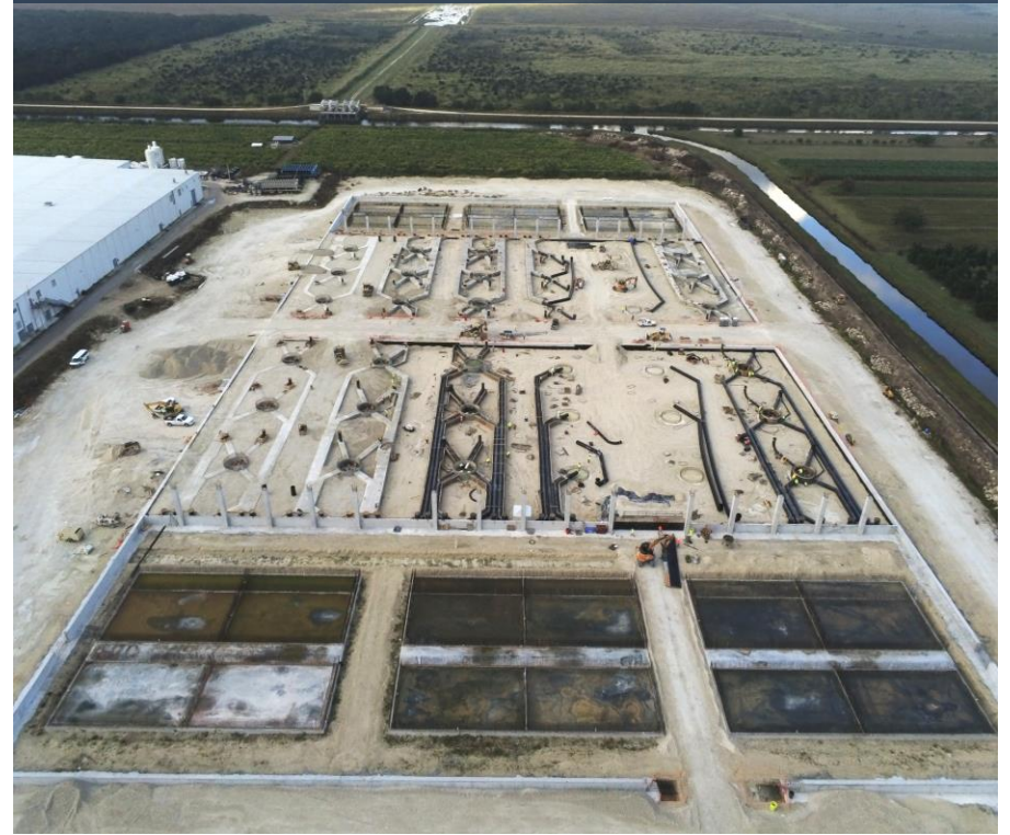
Aerial view of the construction site (Dec '21)
