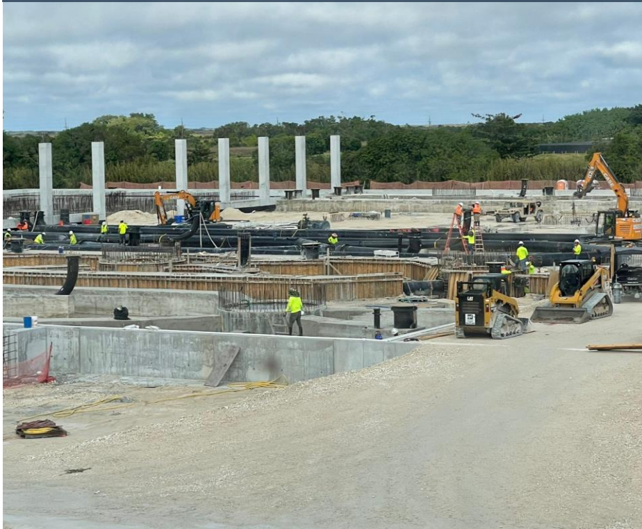
Phase 2 construction activity (Nov '21)
