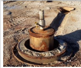
MF-4 saline intake well
