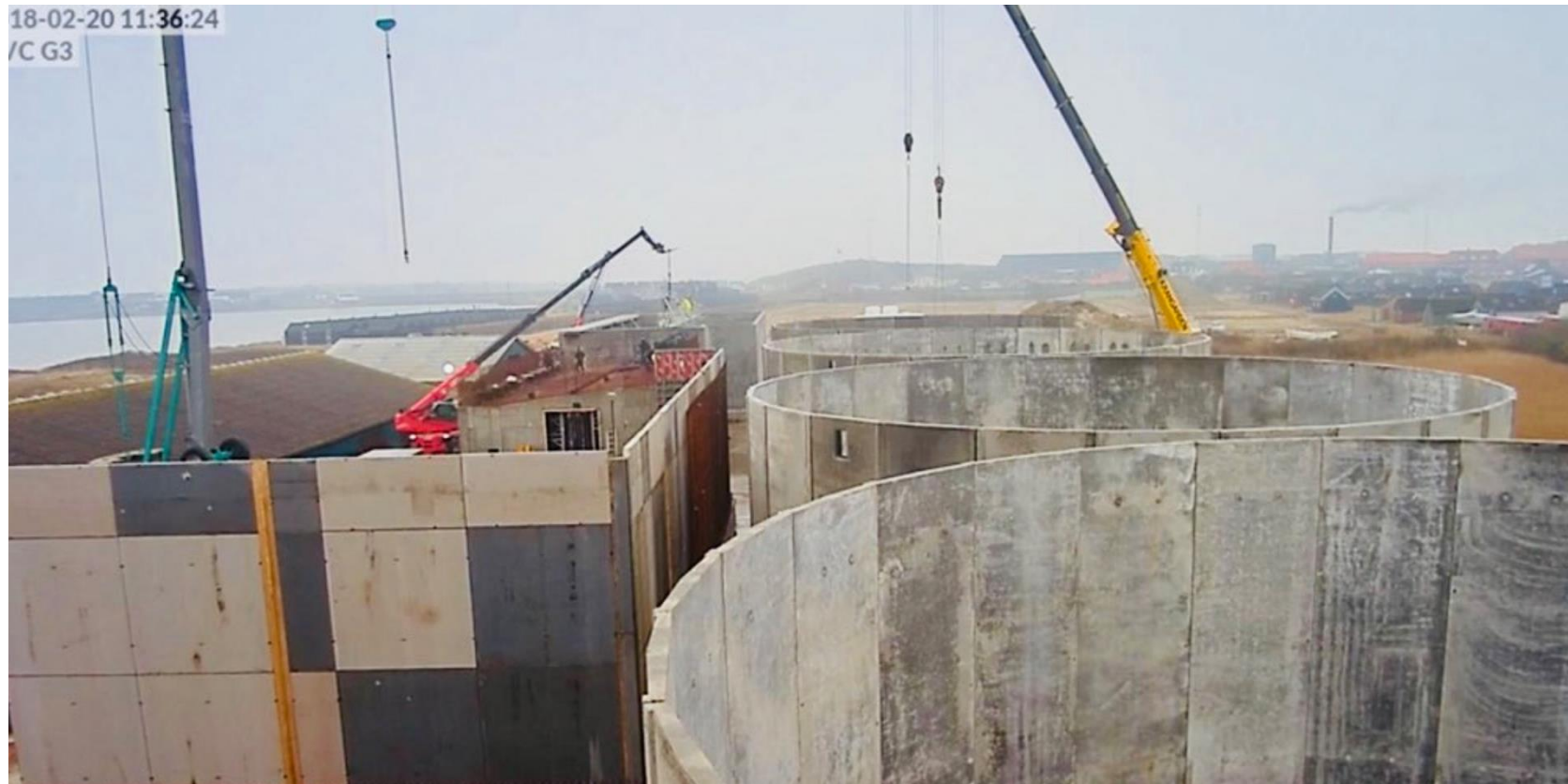
Grow-Out Tanks And Bio-Filters
