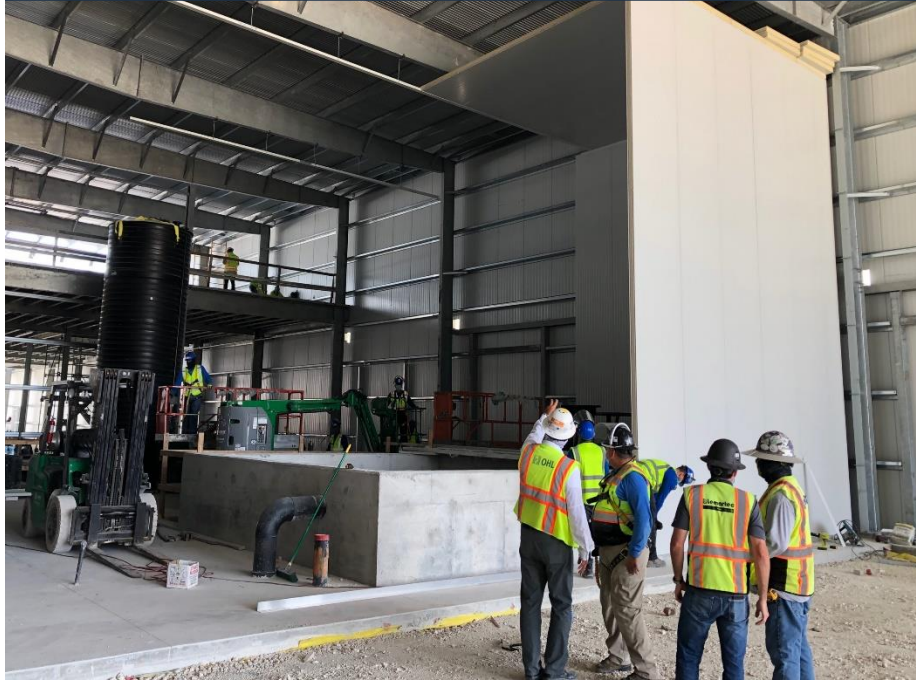
Processing plant under construction
