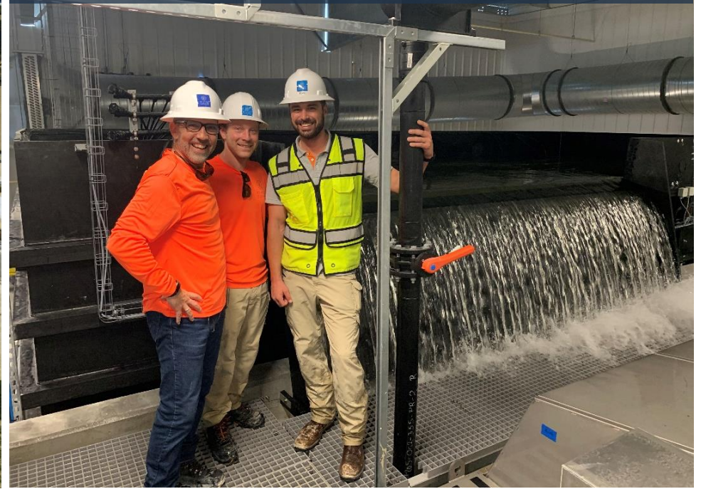
Team members working on commissioning
